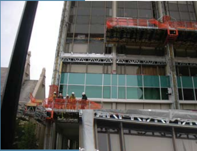
VISION GLASS ON 2/SPANDREL ON THIRD FLOOR
