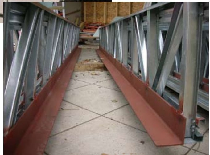
AEGIS COLD-FORMED TRUSSES PROVIDED THE STRUCTURAL FRAMEWORK FOR THE NEW FACDE
