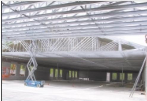
Another inherent advantage of the Ultra-Span system is the relative ease of connections. All Aegis truss shapes are designed to work together. Therefore, smaller trusses and jacks that are built with the standard USC product line can be easily connected to larger USD trusses without elaborate or expensive connectors. As with other Ultra-Span trusses, most
