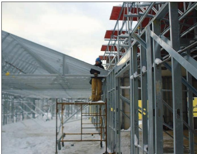
pre-fabricated light gauge system. They offer the easiest, most efficient means for general contractors and framing sub-contractors to procure trusses (and installation services) when the specification calls for light gauge.
