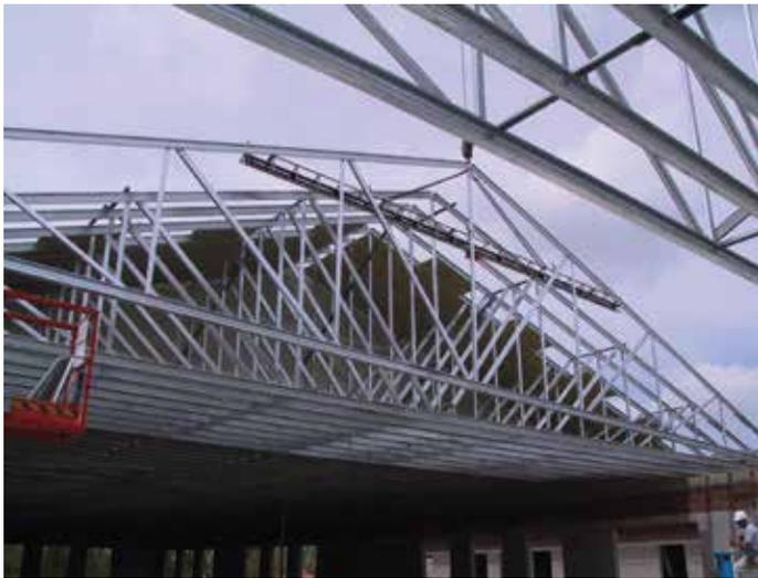
Figure 2. Example use of spreader bar.
