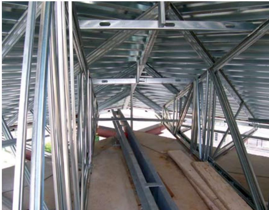
As seen in the photo, a corner girder could not be placed directly at the ridgeline of the Conference Center towers because of large window-cleaning booms that were placed at the corners.
